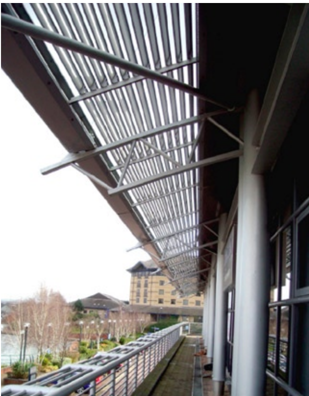
Figure 1 A typical 'brise soleil' installation
